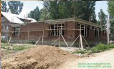
Construction of Community Hall at Patherpora Srinagar
