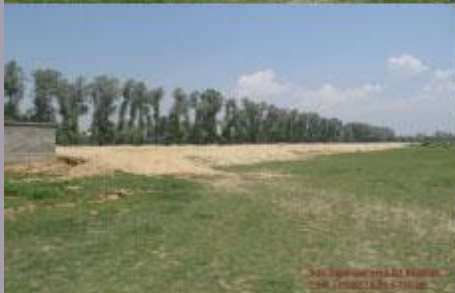
Construction of Community Hall at Patherpora Srinagar
