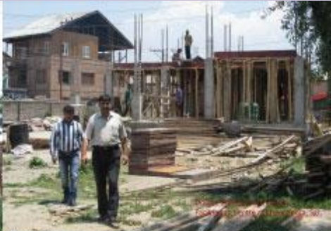
Construction of Community Hall at
