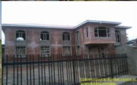
Construction of Community Hall at Patherpora Srinagar
