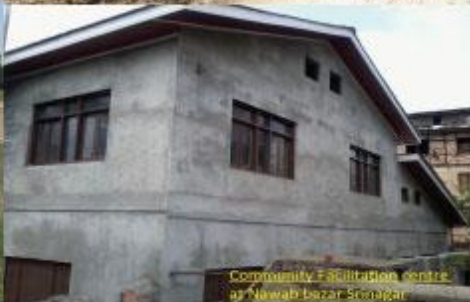
Community Facilitation Centre at Newab Bazar Srinagar
