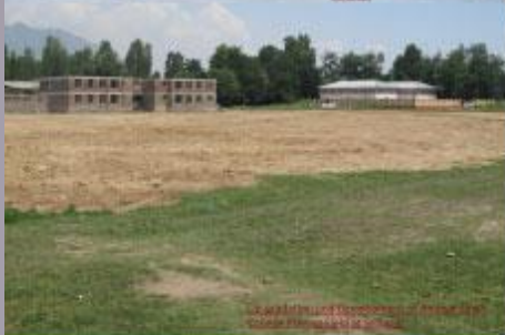
Construction of Community Hall at Patherpora Srinagar
